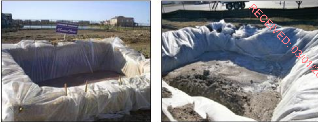
Plate 3-1 Typical concrete wash out areas
