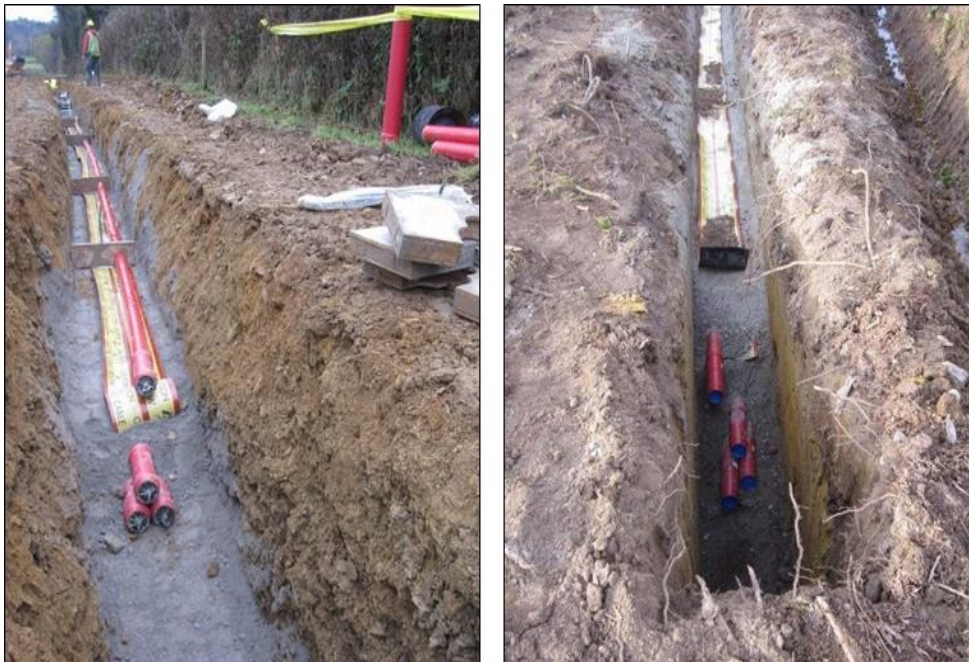
Plate 2-1 Typical Cable Trench View
